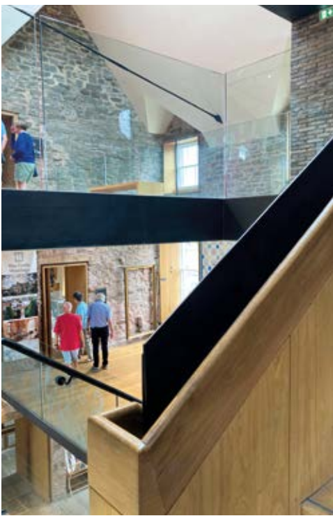
10, 11 Ground-floor entrance space before and after the installation of security reception desk, not envisaged in the original brief. 12-14 The day-lit, three-storey volume with layers of gallery space inserted, reached via a discrete lift and a boldly expressed monolithic steel staircase, which appears to float in the space, with a sheathed and layered balustrade that is stripped away as it ascends the building. The balustrades become fully glazed as they reach the top floor. A minimal steel-tied new roof structure encloses the volume.
