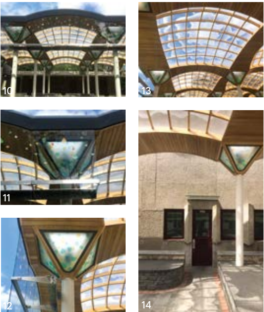
10-12 Details of the vertical glazing to the southern elevation. 13 Cloud-like imagery baked into the thermo-formed solid polycarbonate enclosures to the 'handkerchief' vaults. 14 Original window converted into a door to ease the flow of those leaving the chapel.
